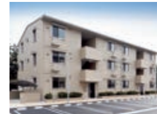
New company housing (Befu)
