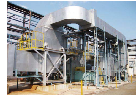
Low NOx boiler (city-gas specifications) (Befu Works)
