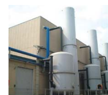
High purity gas generation facility
