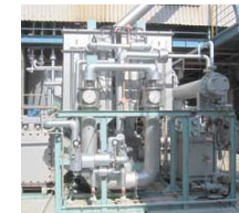
VOC recovery unit (Himeji Works)
