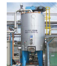
Sludge dryer (Himeji Works)
