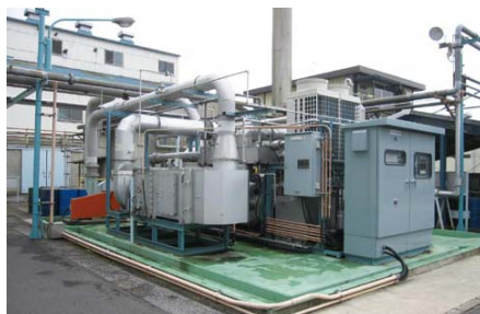
Solvent recovery unit (Chiba Works)
