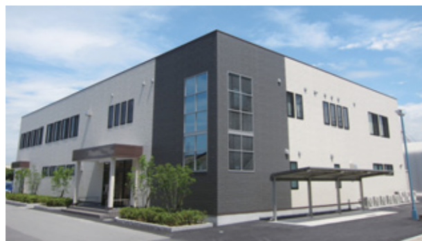
The welfare building equipped with energy-saving LED for lighting
