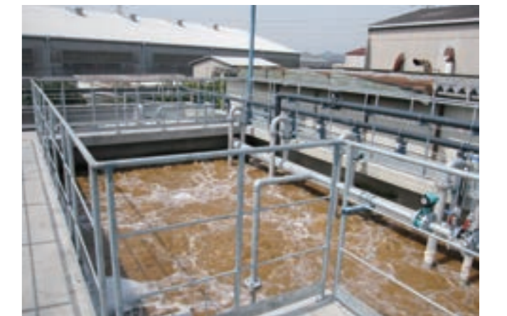
Effluent treatment facility
