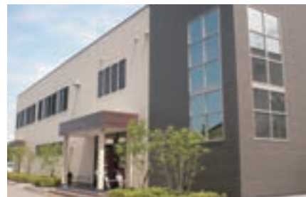
New welfare building at Himeji Works
