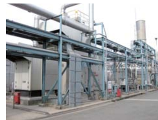
Co-generation facility at Himeji Works
