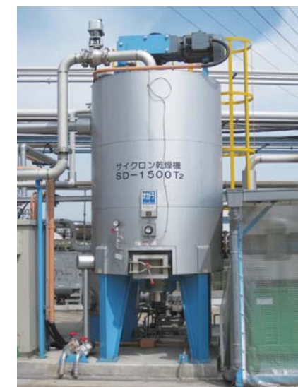
Sludge dehydration facility
