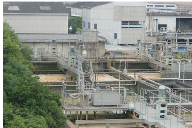
Wastewater treatment facility
