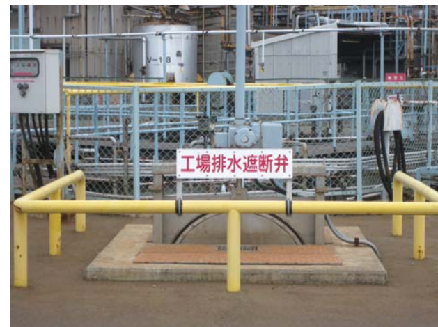
Emergency shut-off valve at Befu Works
