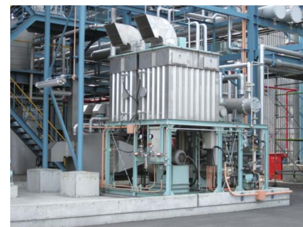
VOC recovery unit
