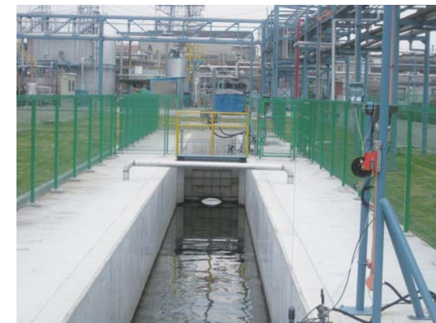
Emergency shut-off valve at Himeji Works
