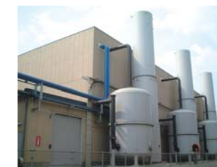
High purity gas generation facility
