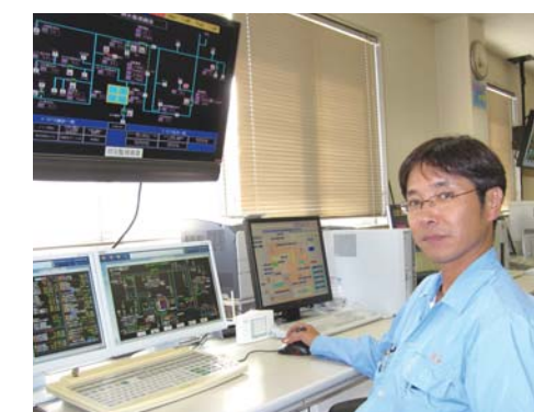
Furutani Hideki Safety, Environment and Utilities Dept., Befu Works
