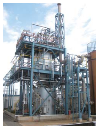
Submerged combustion-type waste liquid incinerator
