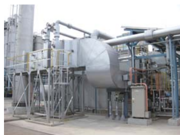
Low NOx boiler using city gas
