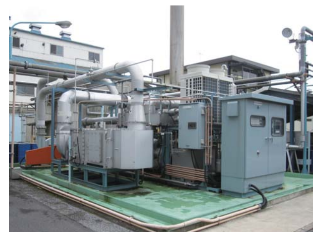
Solvent recovery unit (Chiba Works)
