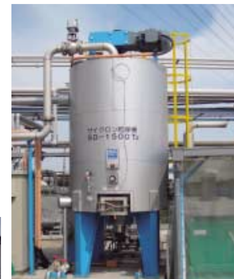
Sludge dehydration facility
