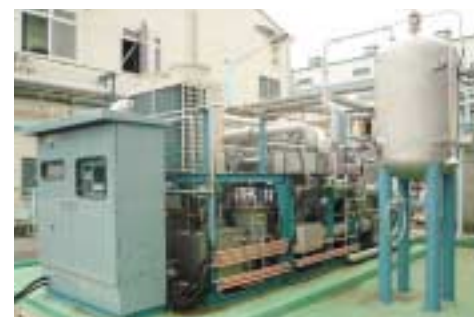
Adsorption recovery facility (Chiba Works)
