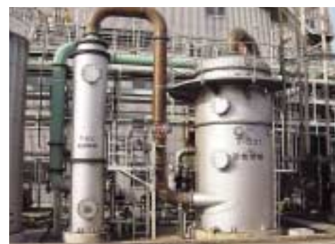
Exhaust gas pollutant removal equipment (Befu Works)
