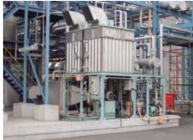
Volatile organic compound (VOC) recovery facility
