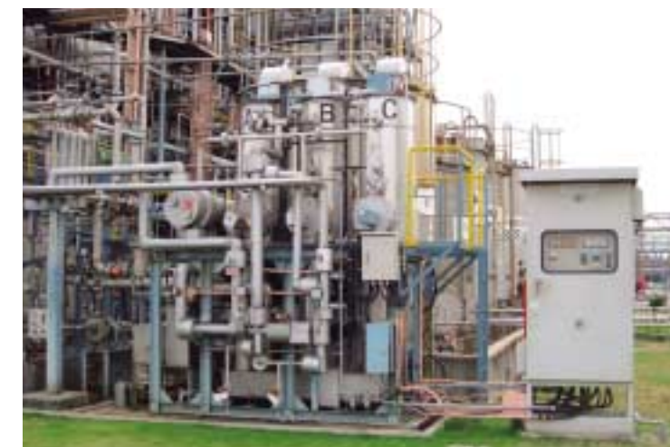
Gas recovery facility (Himeji Works)
