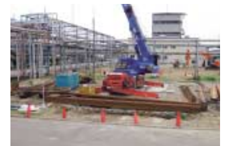
Installation of emergency shutoff valve under way at Himeji Works
