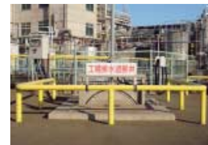
Emergency shutoff valve at Befu Works
