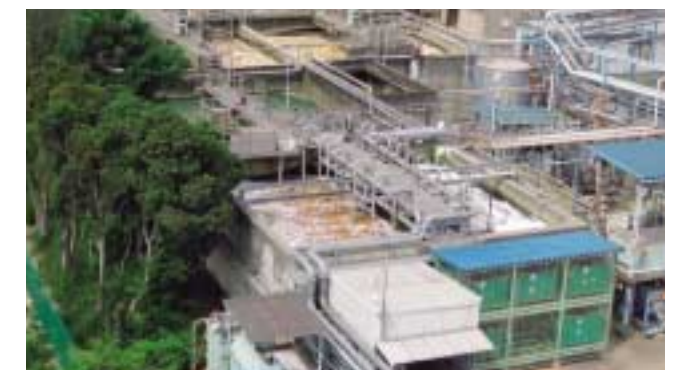
Wastewater treatment facility
