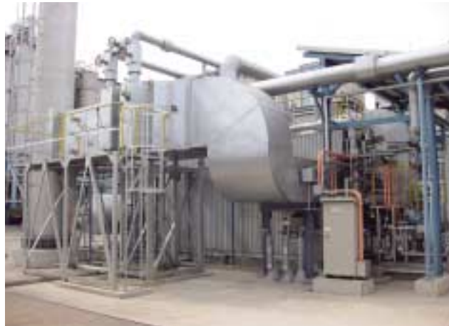
Low NOx boiler using city gas
