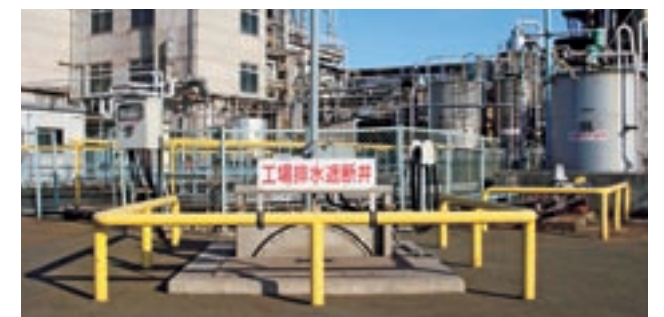
Wastewater treatment facility (Befu Works)
