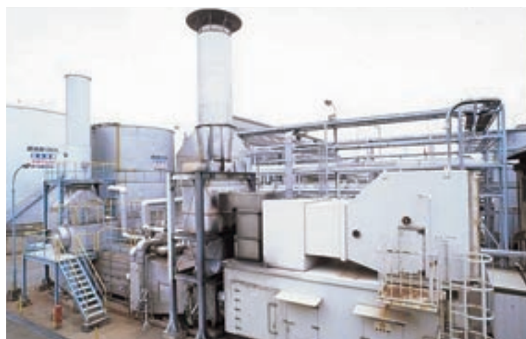
This cogeneration facility also contributes to reducing the amounts of SOx and particulate matter (Befu Works)
