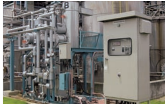
Gas recovery facility (Himeji Works)
