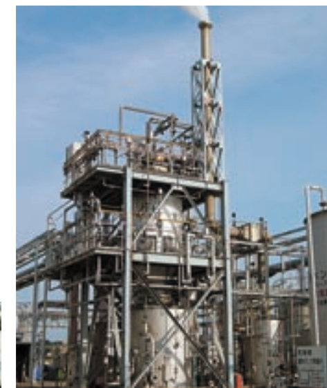
Waste-incinerating volume-reduction plant
