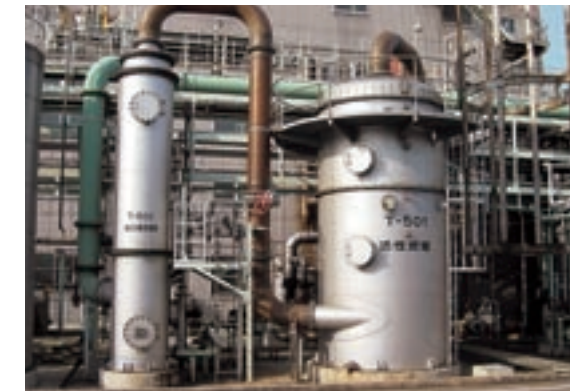
Exhaust gas pollutant removal equipment
