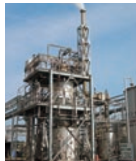
Waste-incinerating volume-reduction plant
