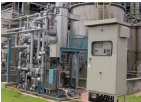
Gas recovery facility (Himeji Works)
