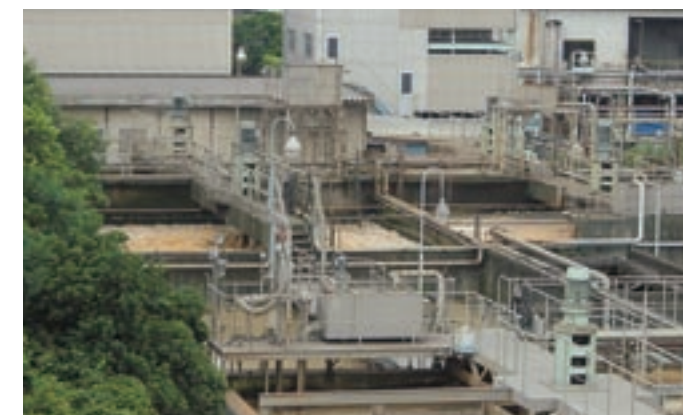
Wastewater treatment facility (Himeji Works)
