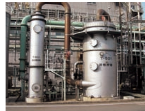
Exhaust gas pollutant removal equipment
