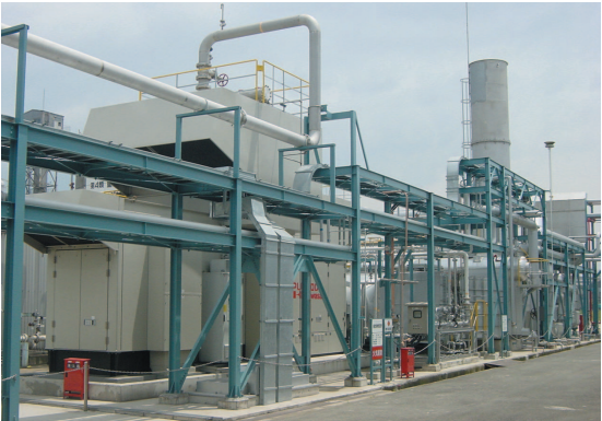
Introduction of a cogeneration system (Himeji Works)
